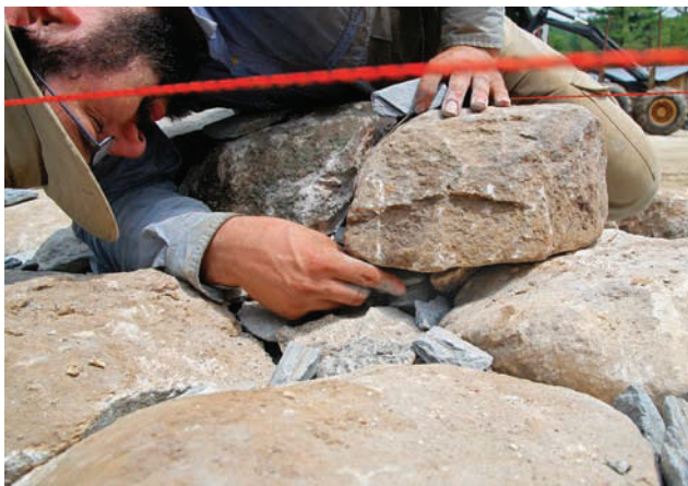
Pin from within. Pinning stones shim the face stones level and solidify their placement. Never pin from the face of the wall because it will just fall out over time.
