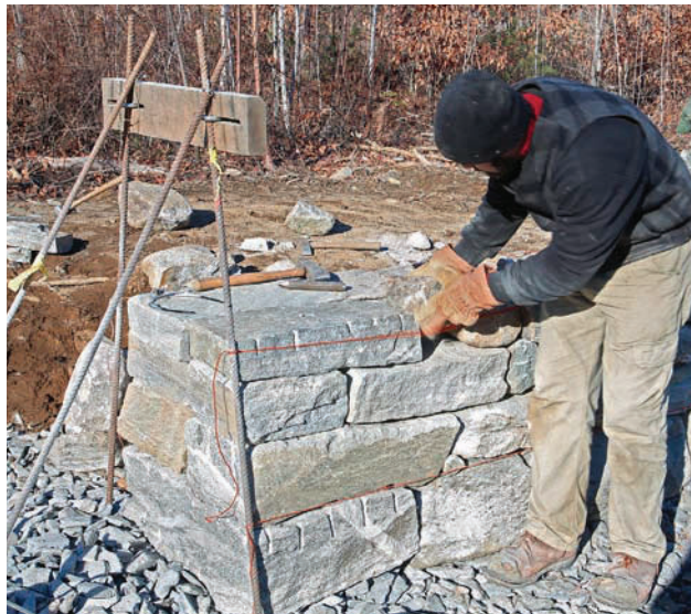
Build ends and corners like log cabins. Shaping is often needed to fit end stones. Alternate stones that span the wall width with long stones that tie back into each course.
